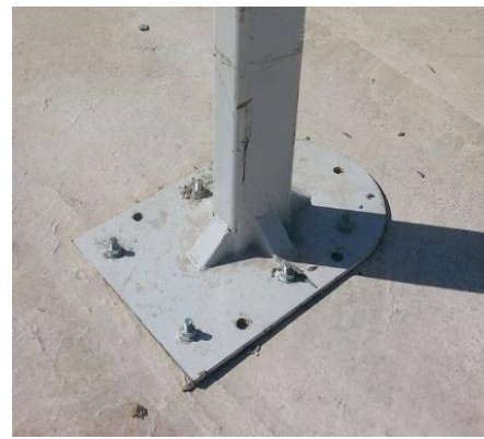
Figure 4. Bridge floor concrete and base plate connection
