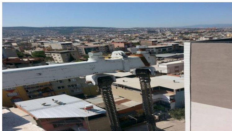
Figure 5. The chain attaching the platform to suspension leg
